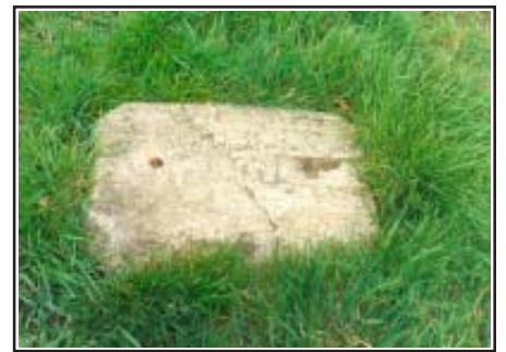
Concrete sleeper at Congresbury Used due to a wartime shortage of timber. Spring 1990
