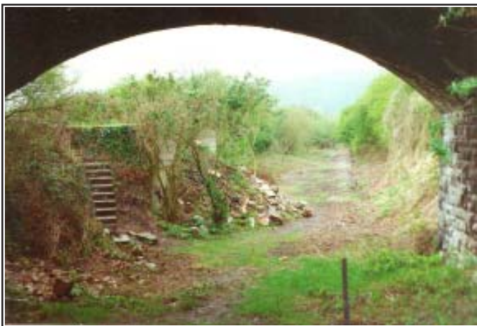
Early days of cycleway at Cheddar showing steps down fro loading platform.
